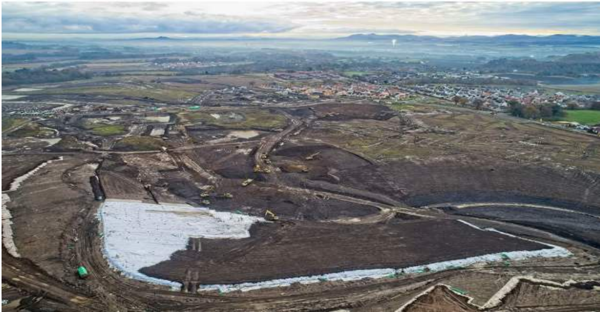
Site under remediation (courtesy of I&H Brown)
