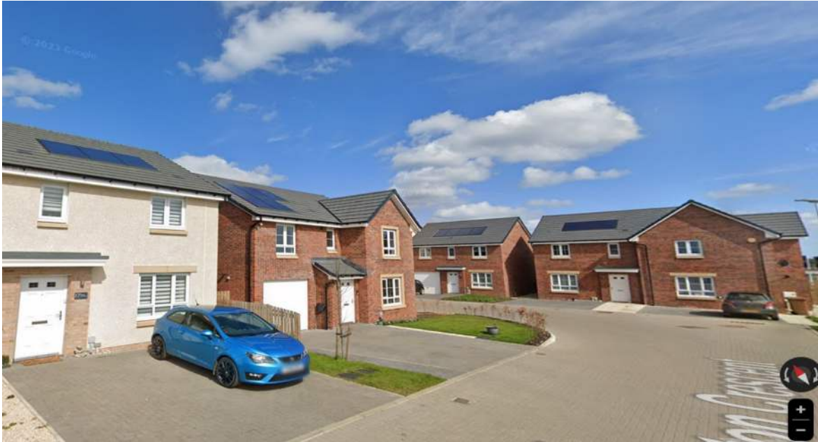
Barratt Development where red brick has been used to pick out a junction point.
