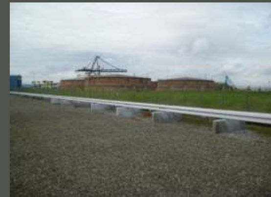
Underground tank storage= 7/120
